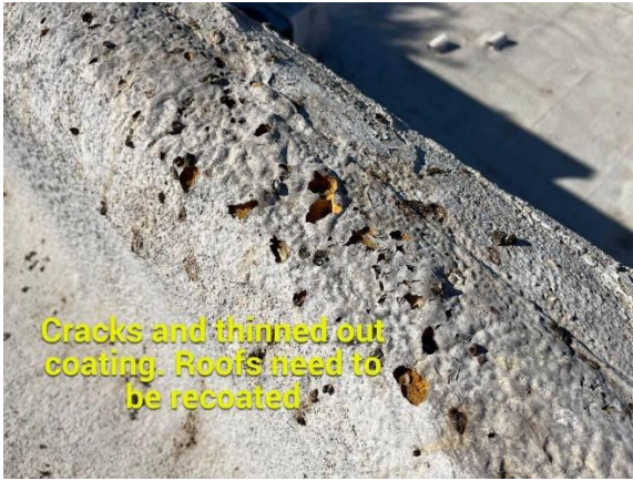
Cracks and thinned out coating. Roofs need to be recoated
