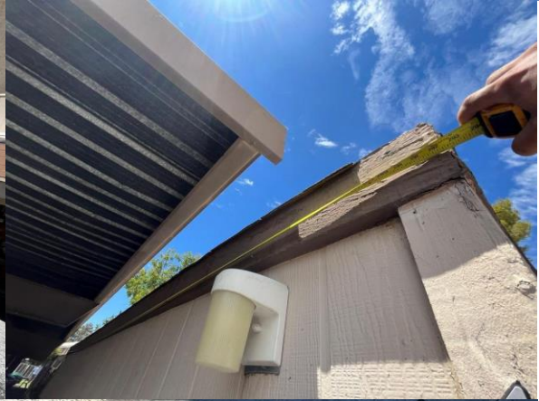
Heavy granule loss and loose shingles.
